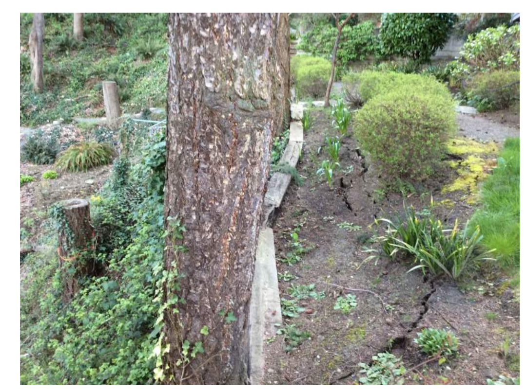
VISIBLE FAILURE OF SLOPE
