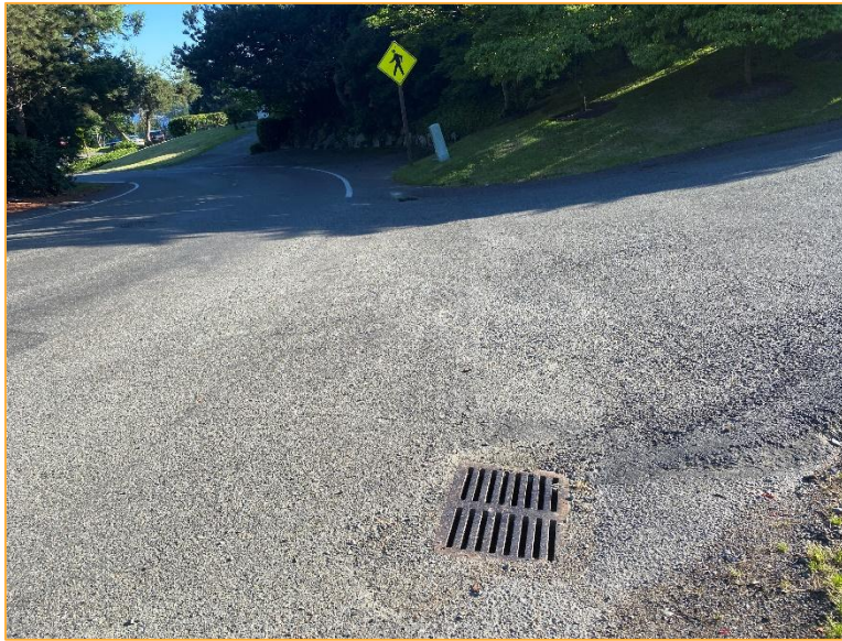
Photo 3 – Facing southeast on the north corner of Mercerwood and SE 43 rd PI. Runoff enters a catch basin and continues southwest.
