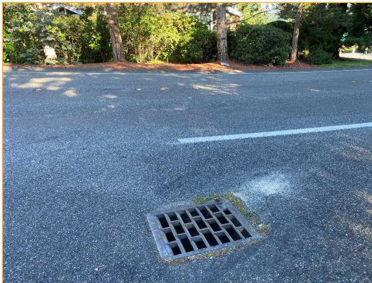
Photo 4 – Facing east on the south corner of Mercerwood and SE 43 rd PI. Runoff enters a catch basin and continues east.
