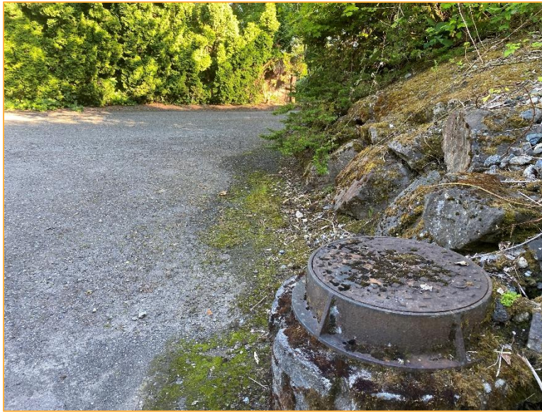
Photo 7 – Facing southeast along the north side of 100 th Ave SE. Runoff is conveyed to a catch basin and continues southeast.
