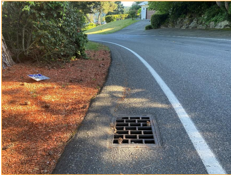
Photo 5 – Facing east side of Mercerwood. Runoff enters a catch basin and continues southeast.
