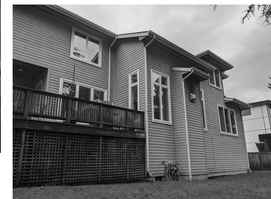
BUILDING VIEW - EAST
