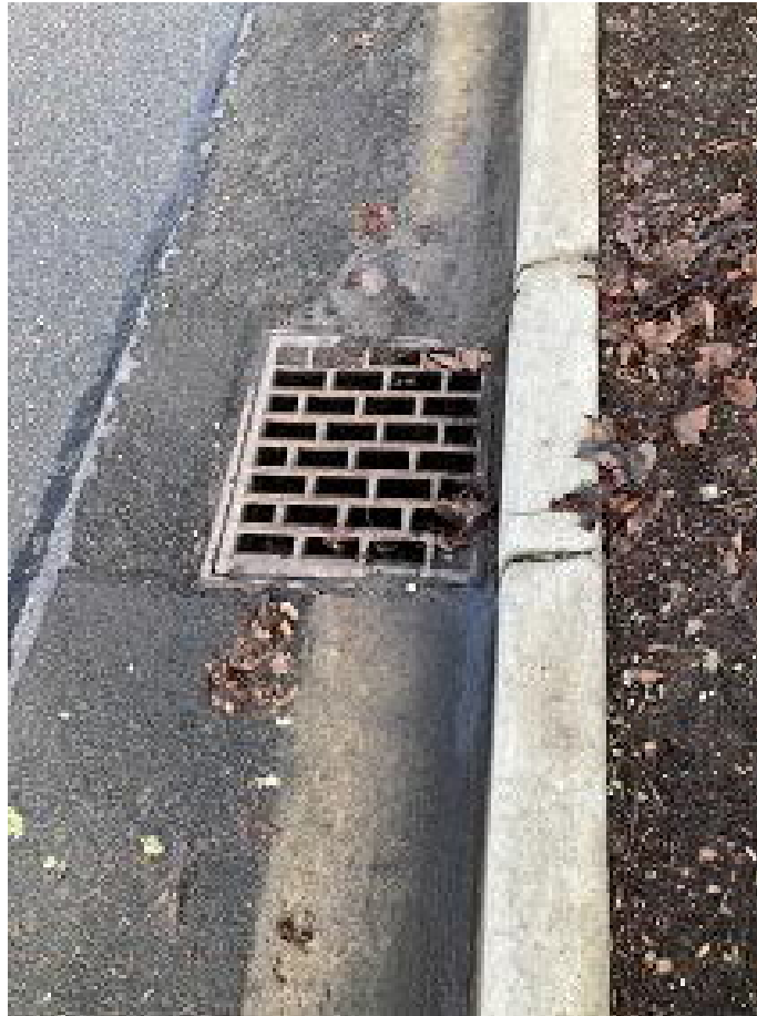
Picture 16: West Mercer Way just northeast of the I-90 on-ramp End of ¼-mile analysis; from here pipes cross west (left of page) under W. Mercer Way 18" SD WSDOT OWNED PIPE
