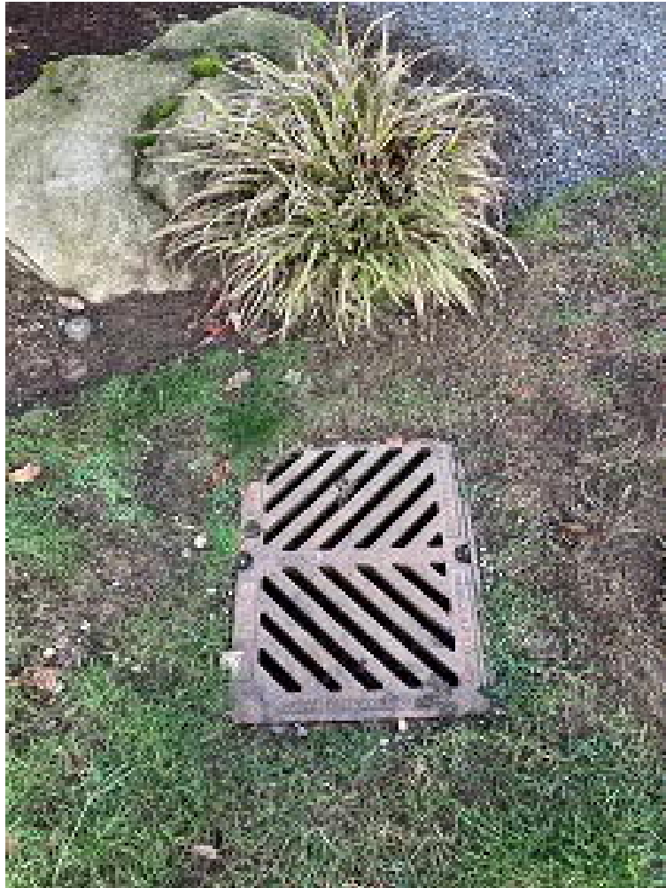
Picture 4: ROW in front of 2227/2223 71 st Avenue SE flowing north 12" SD
