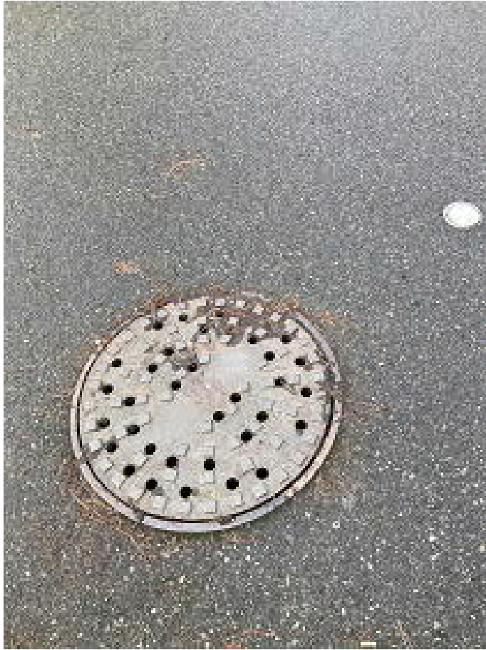
Picture 10: In the street in front of 2212 66 th Avenue SE From here, the storm pipes go northwest into Aubrey Davis Park 18" SD WSDOT OWNED PIPE
