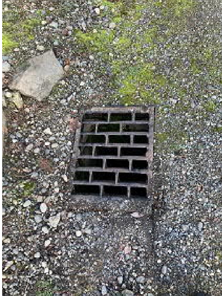
Picture 5: ROW in front of 2215 71 st Avenue SE 12" SD
