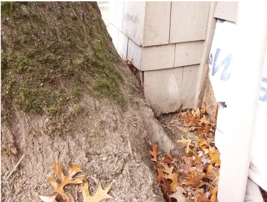
Figure 6. Looking NW at the base of the large oak pressing into the side of the garage. Note where the soil was removed to expose the roots in this area.
