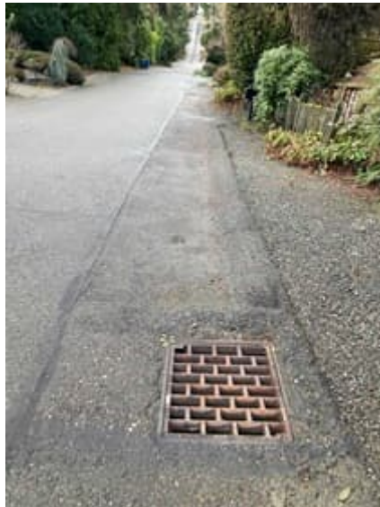
Picture 16: North ROW in front of 6824 SE 32 nd Street (looking west) Type 2 catch basin. See the next two catch basins downstream of this one.
