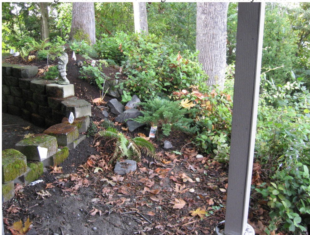
New retaining wall to tie in with existing wall northeast of subject trees
