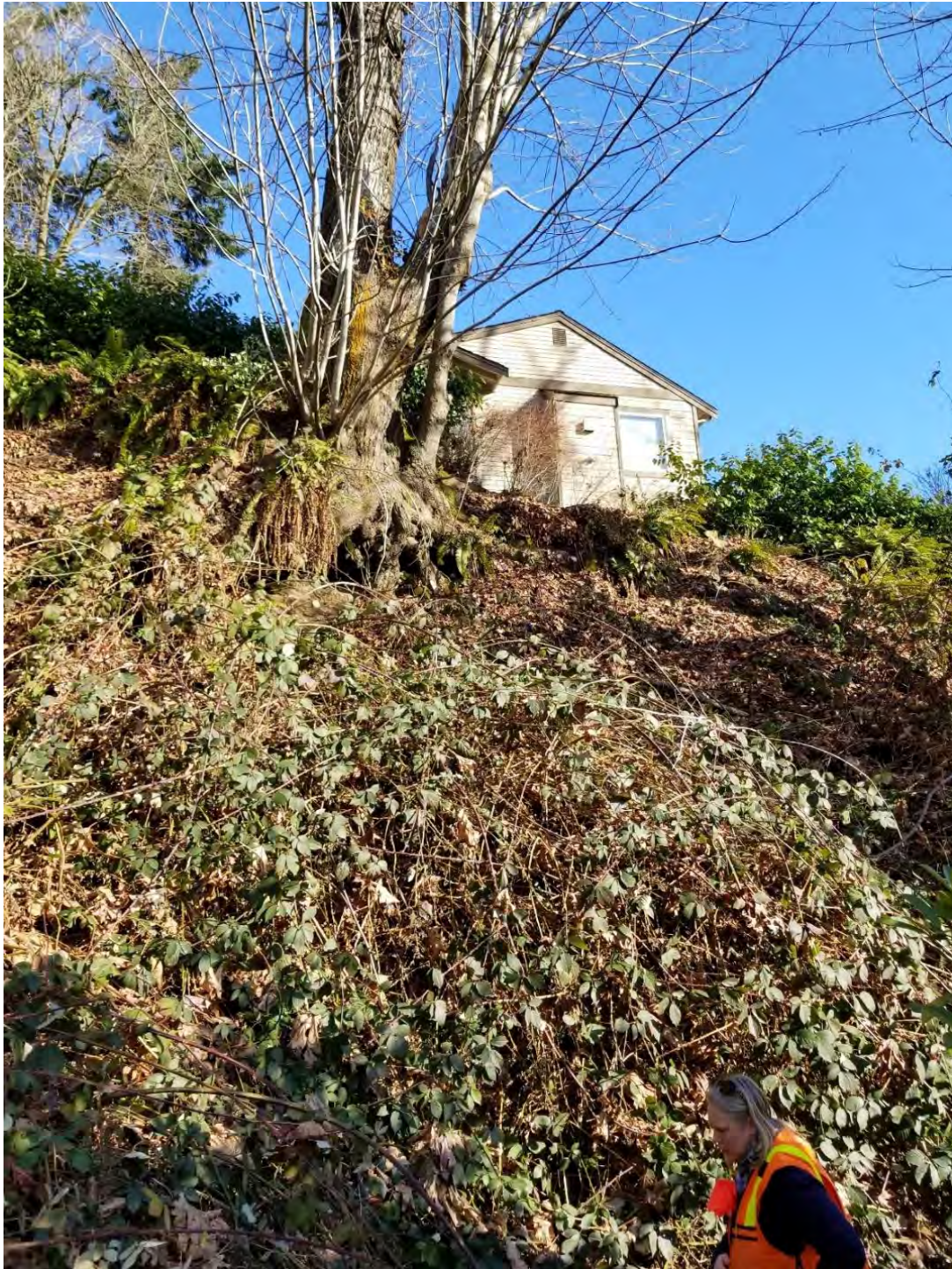
Photo 1—Steep slope to north of stream channel.
