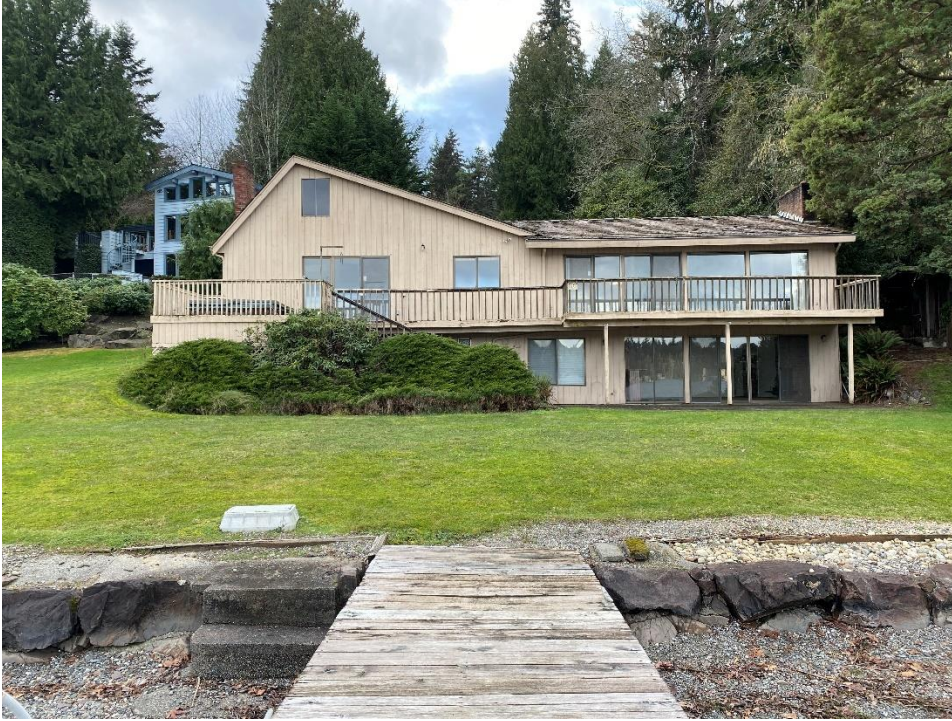
Existing house, view from existing dock.
