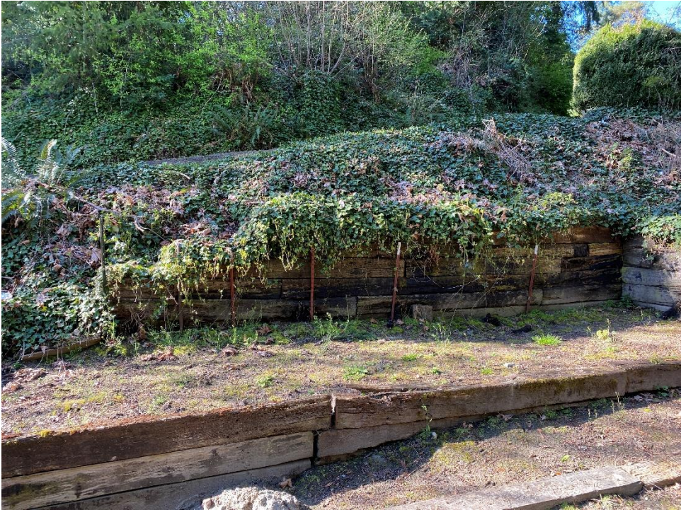
View from west of garage, looking south. Yielding timber retaining wall along south property line
