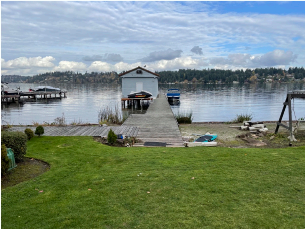
Photo 1 - Existing dock looking waterward.
