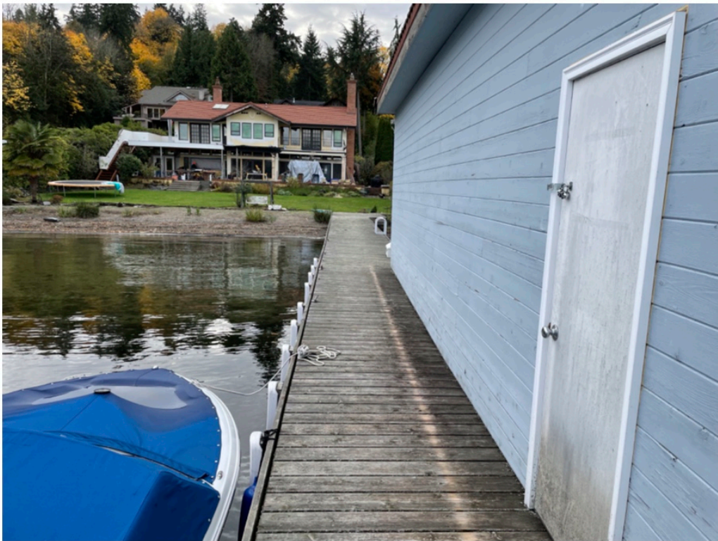
Photo 2 - Existing dock looking landward.
