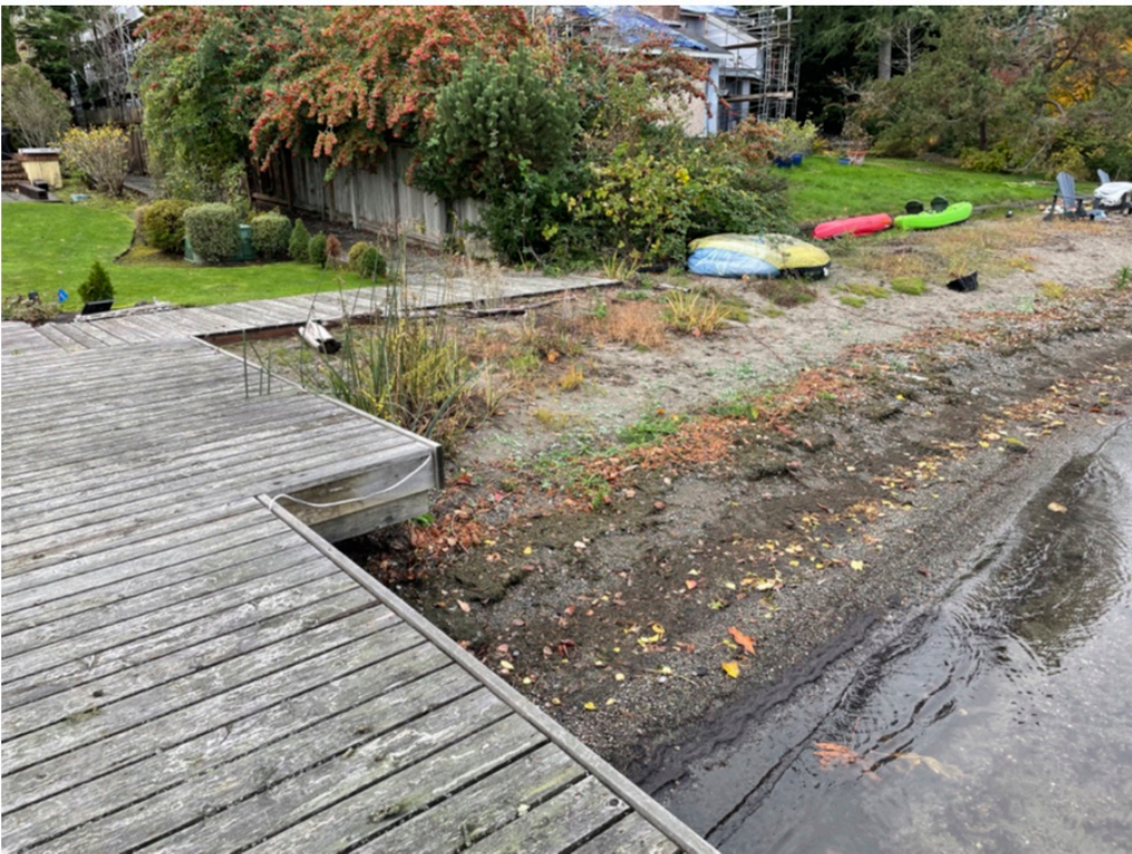
Photo 4 - Shoreline conditions looking West.
