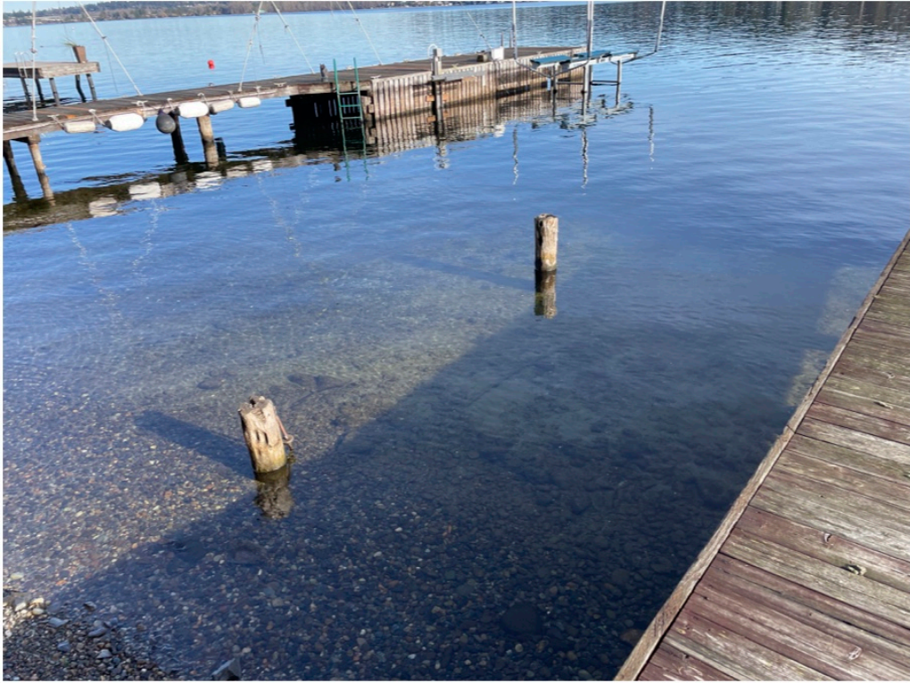
Photo 7 - Two mooring piles to be removed.
