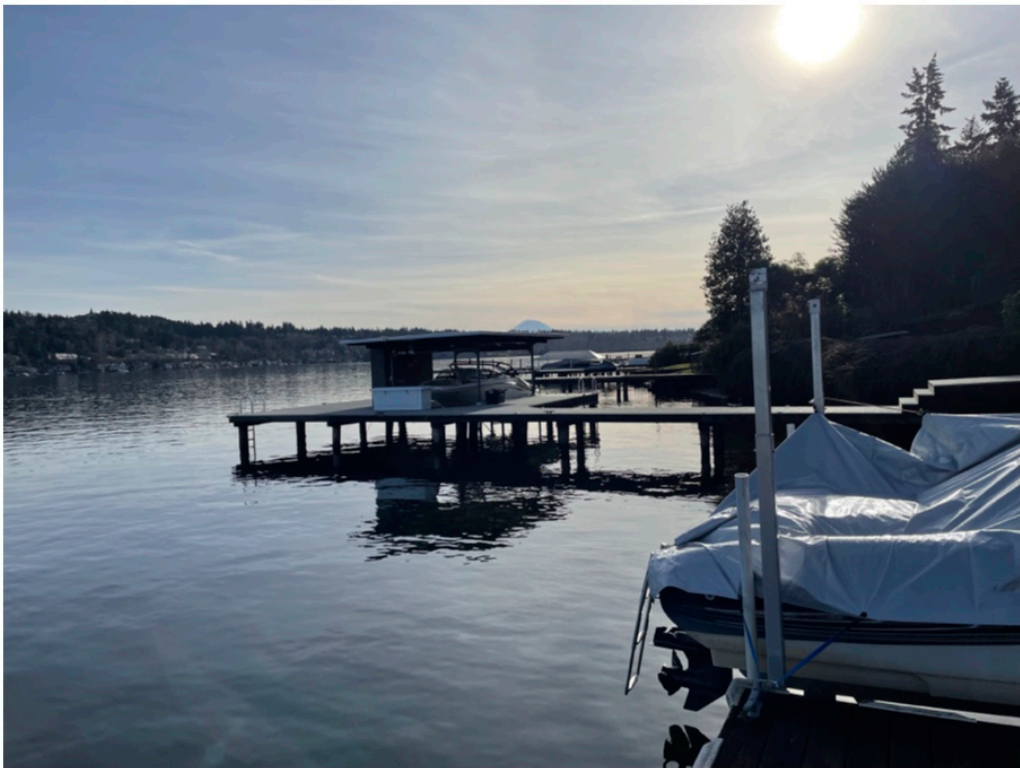
Photo 6 - Shoreline condition south of the project.
