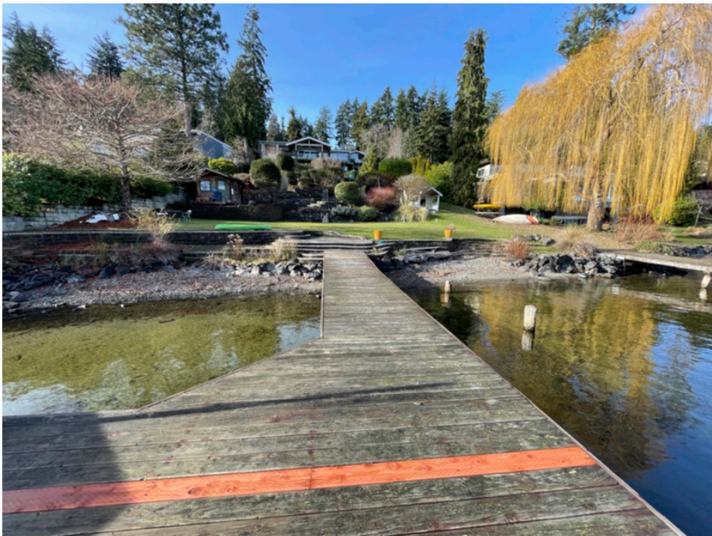
Photo 2 - Existing dock looking landward.
