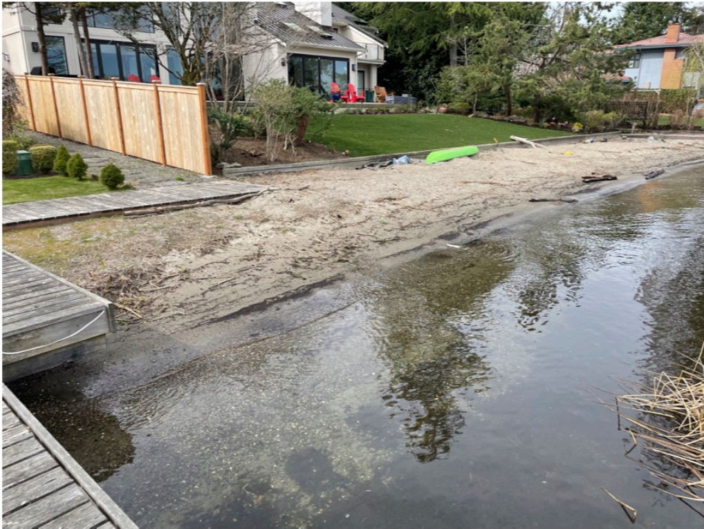
Photo 3 - Existing shoreline conditions at the site looking west.
