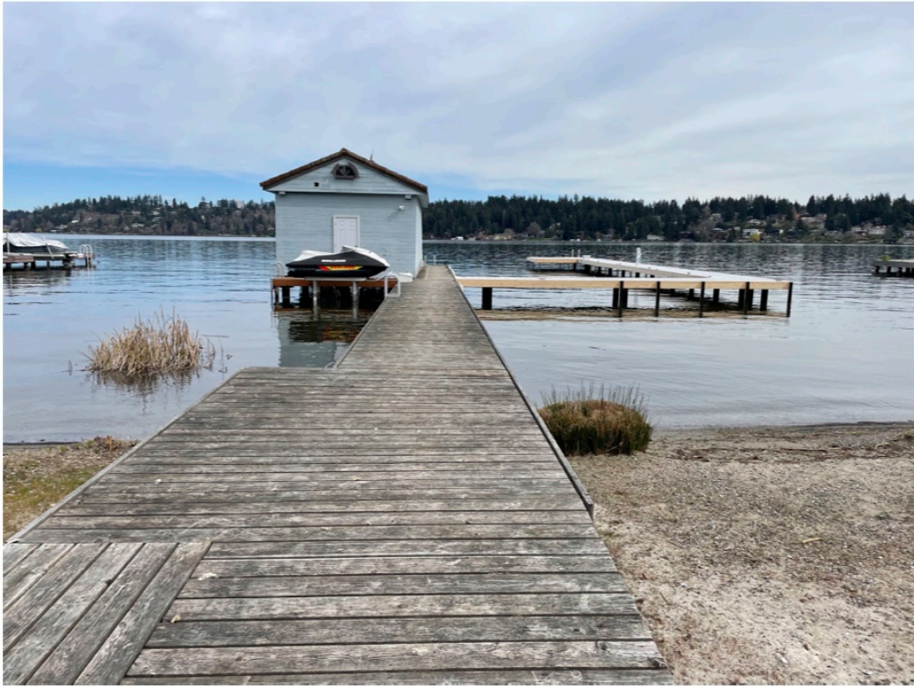
Photo 1 - Existing conditions looking waterward.
