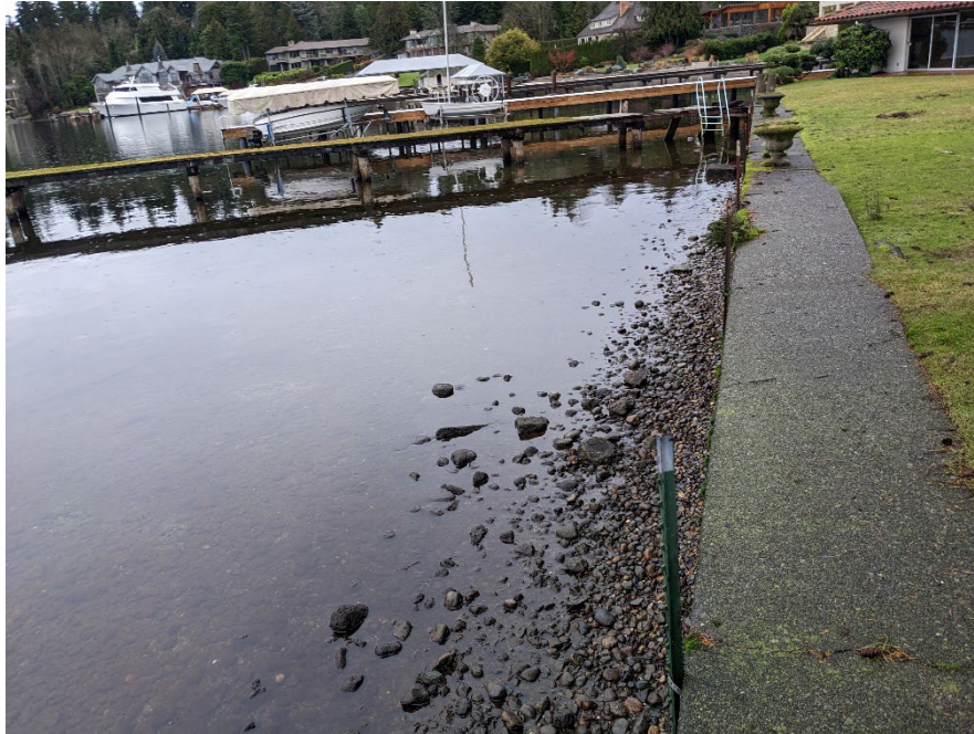
Photo 1. View of bulkhead along shoreline in subject property.
