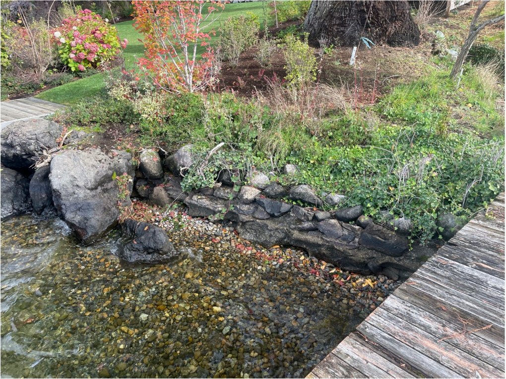
Photo 3 - Existing shoreline north of dock.
