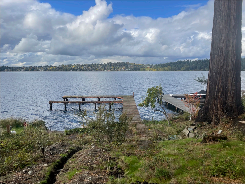
Photo 1 - Existing dock looking waterward.
