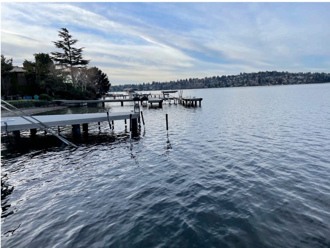
Photo 6 - Existing conditions west of the project.
