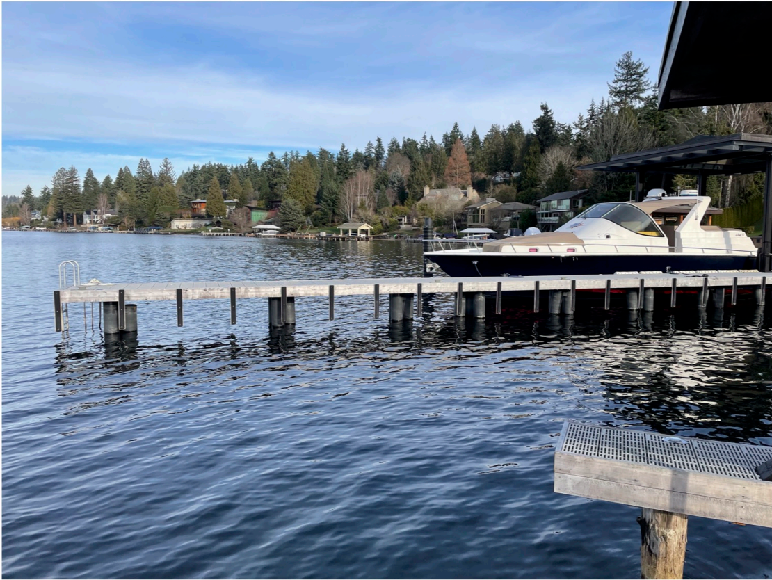
Photo 5 - Existing conditions east of the project.
