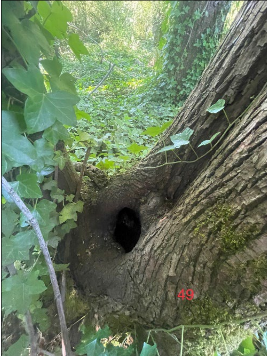
Photo 18. Tree #49 with hollow trunk.
